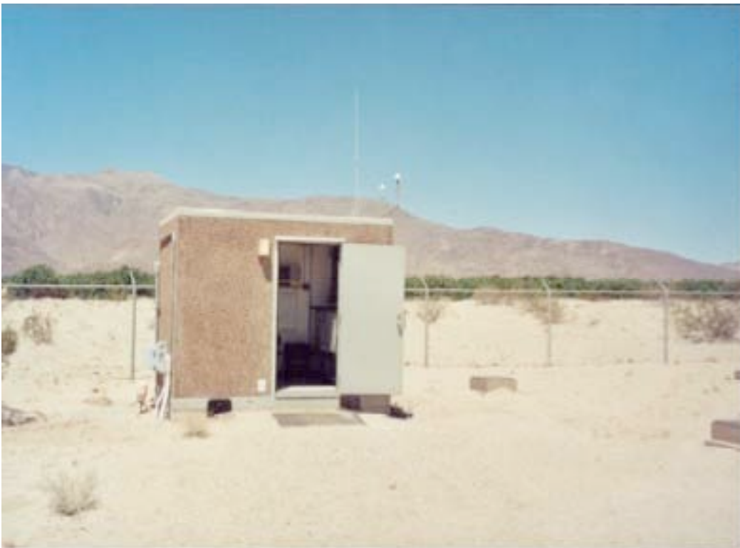
The UCSB Borrego Downhole Array Facility
