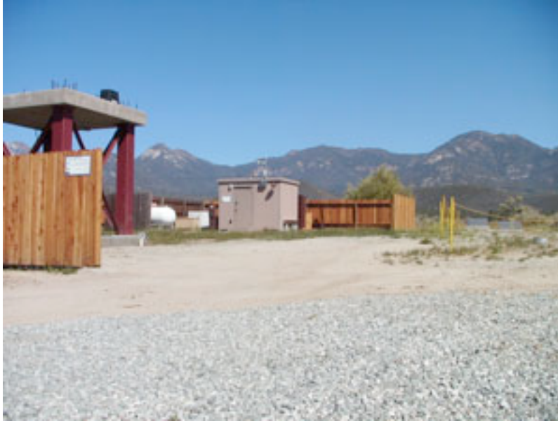
Garner Valley Field Site and SFSI Structure
